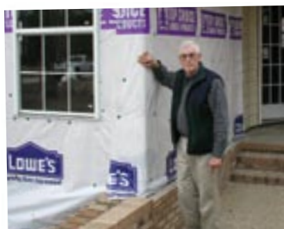
Ed Evans at a home construction site in Biloxi.
